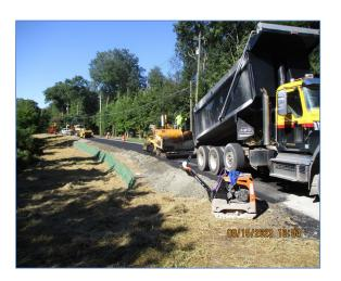
County Road 61 Embankment Repair—GRSS Geo-cell Retaining Wall
