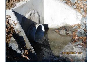
County Road 61 Drainage Repair—No Dig Cure-In-Place Slip Lining
