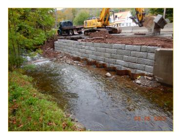
Embankment Restoration at Bridge 115 on CR 123, Rockla (Typical Example-Repair Work Designed/Constructed by DPW)
