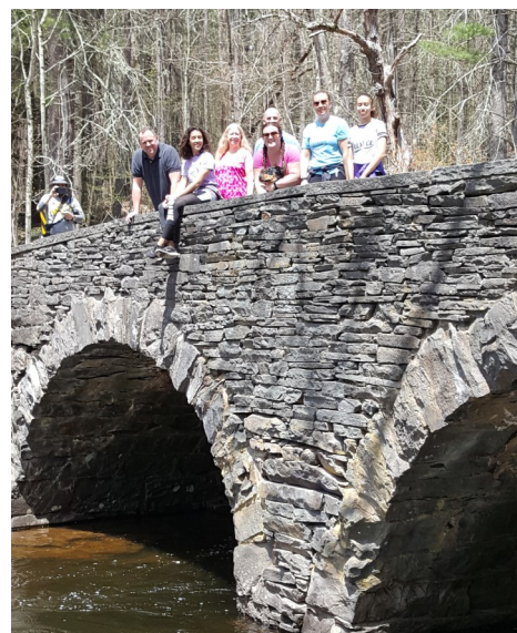
Tusten Stone Arch Bridge, part of May's Tusten Mountain walk.
